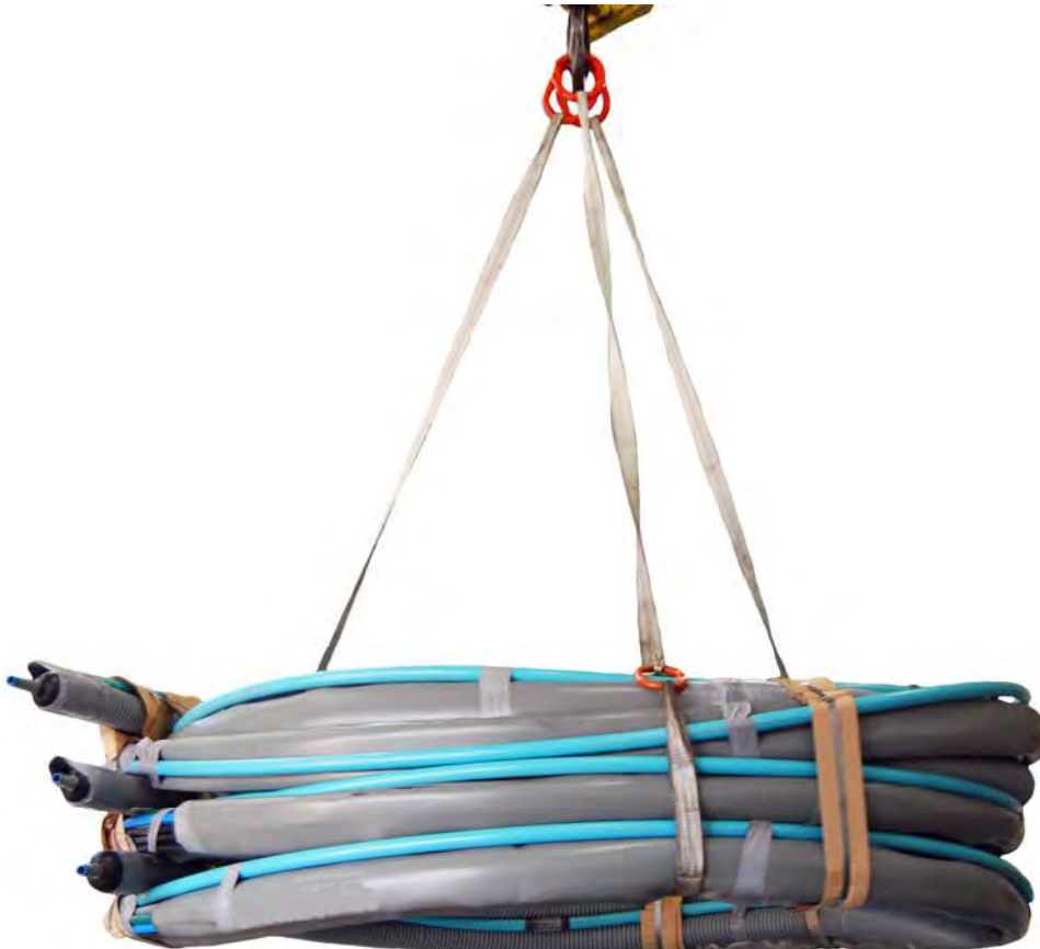
Ground anchors with T-001 27x34 mm valvate tubes
