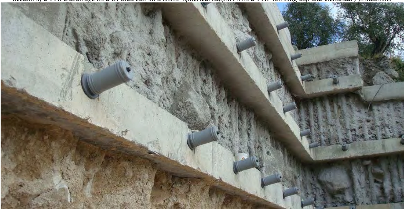
Section of a TTR anchorage on a DI load cell on a DDSF spherical support with a TTR-450 long cap and elementary protections
