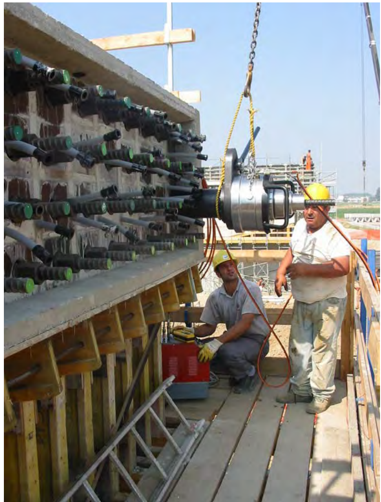
Bar tensioning of diam. 40 mm with DD2000KN jack and TTM250-A pump
