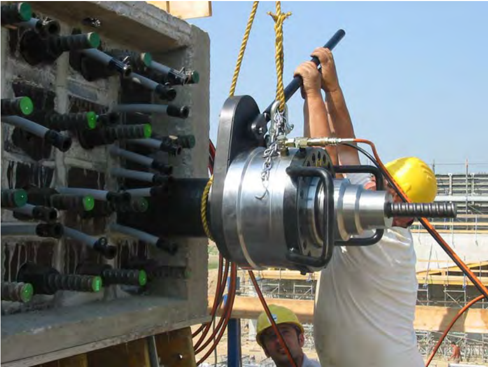
Bar tensioning with DD2000KN jack
