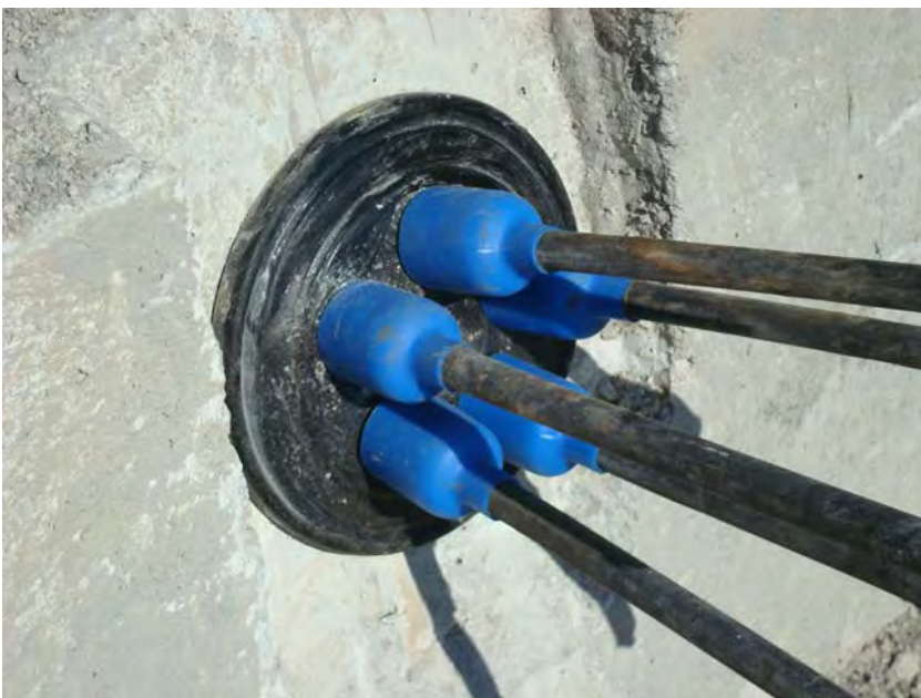
Application of a 5TTR15 anchorage orthogonal to the wall
